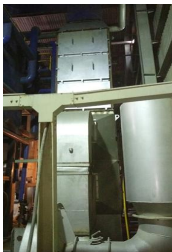
Water economizer in a factory
